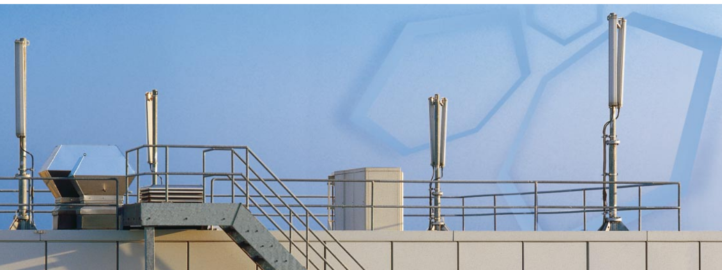
FIG 1 Examples from Rohde & Schwarz BTS antenna program: sector antennas providing coverage in mobile-radio networks
